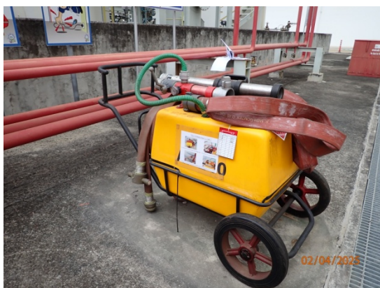
Wheel Foam Chemical Extinguisher
