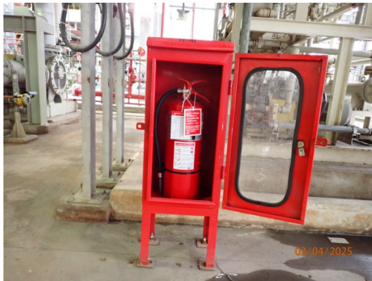
Portable Dry Chemical Extinguisher
