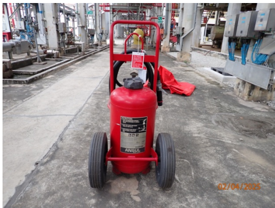
Wheel Dry Chemical Extinguisher
