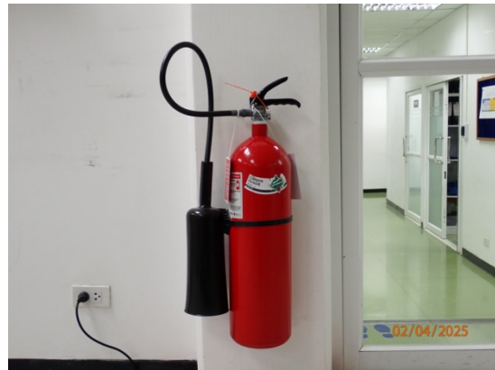
Portable Fire Extinguisher (CO 2 )
